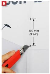
Make 2 small hole in the graphic and one for the cable.
